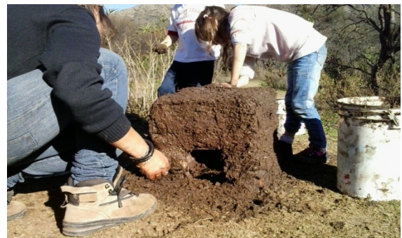
Construction of the rocket-oven for the school.
