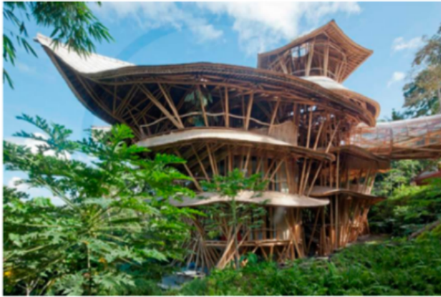
Fig. 5.39 - Green School Bali (Indonesia) por IBUKU architecture
