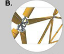
Steel cable running through the joinery to pull the structure in compression
