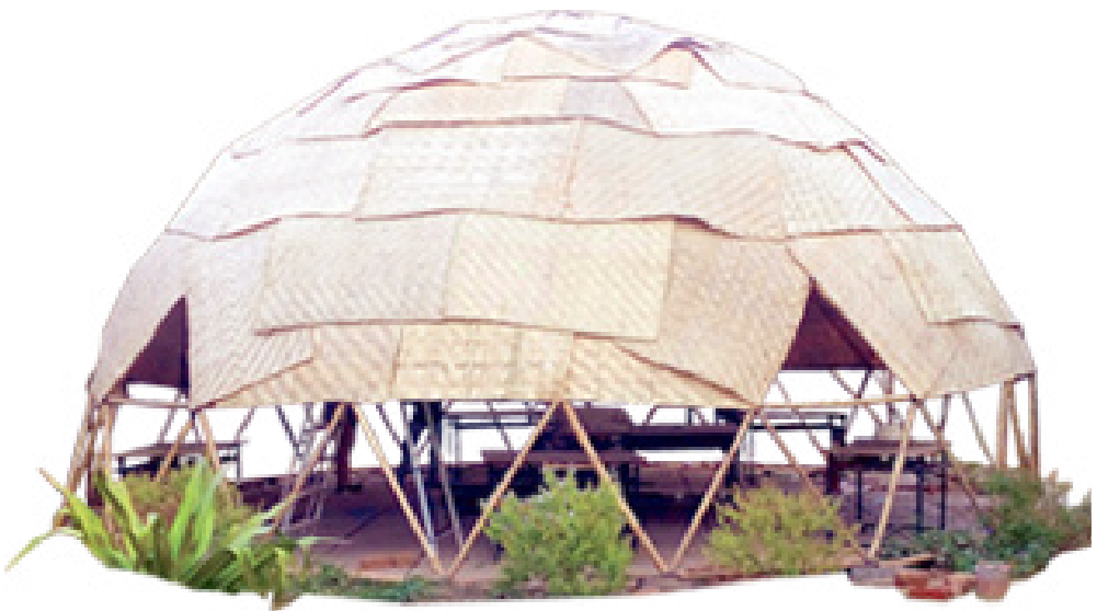
Fig. 5.7, 5.8 - Adaptable Bamboo Geodesic Domes
